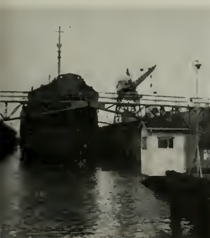
Dock is being raised with vessel secure on blocks. Ship is centered by means of plumb bobs at each end of vessel.
